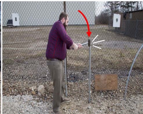
10. Pound Support Posts In Ground With Pipe Pounder & Sledge
