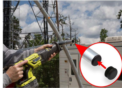
19. Cut Off Excess & Insert End Plug
