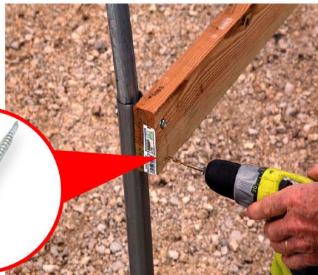
22. Screw Side Rails Into End Post
