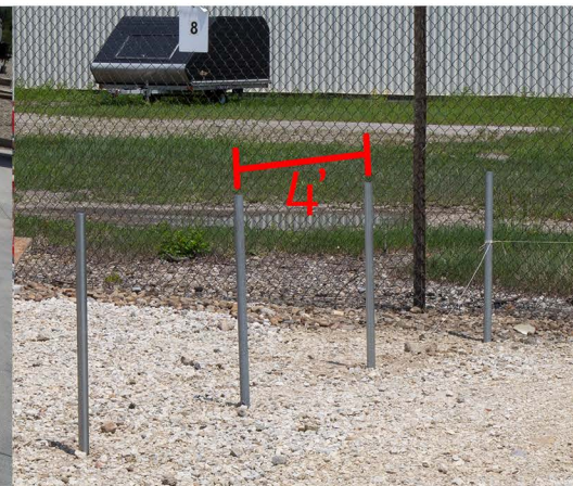
8. Measure & Line Up Support Posts 4' On Center
