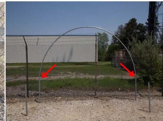
12. Attach The Rest Of The Hoops To Support Posts
