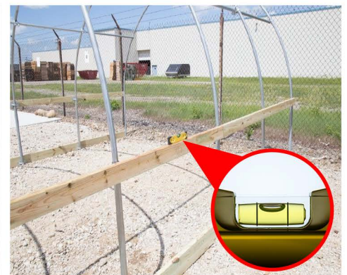
24. Make Sure Side Rails Are Level
