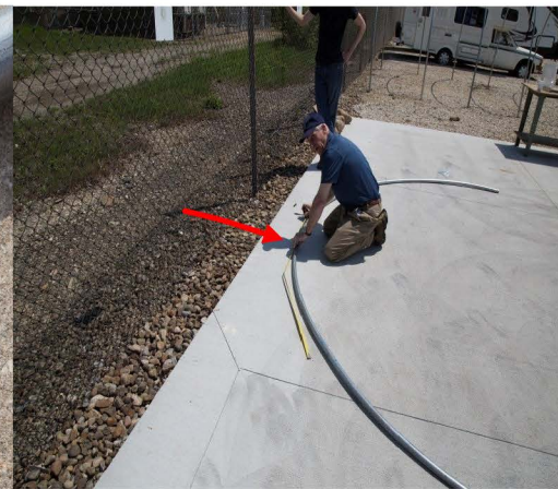
7. Find Center Of Arch And Add Mark
