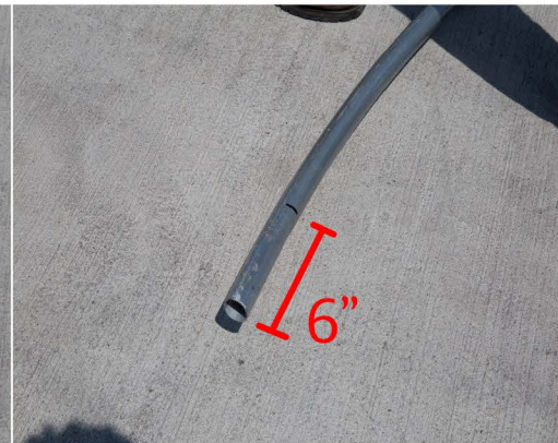
3. Confirm 6" Marks On Support Post
