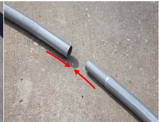
4. Connect Swedge Ends Together
