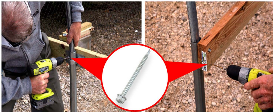
21. Attach Wooden Side Rails
