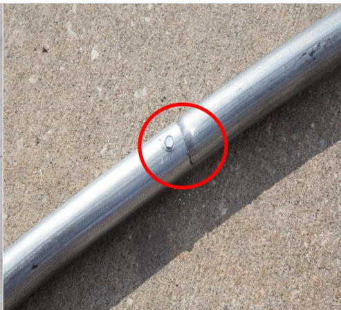
6. Confirm Connected Ends Are Secure
