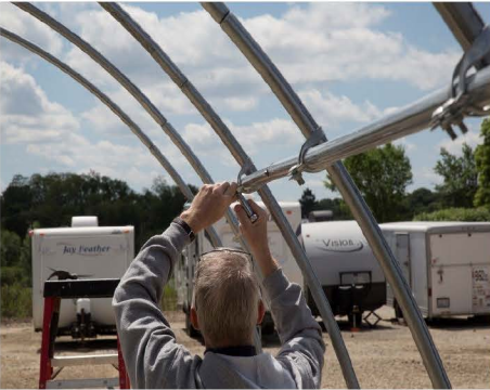
17. Finish Installing Side Braces For Both Sides
