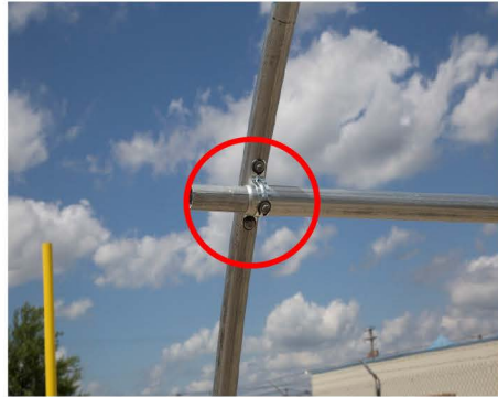
18. Use Pole Strap For Ends Of Side Purlin
