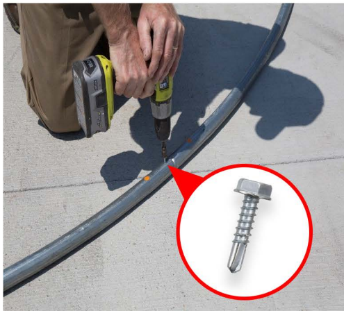
5. Use Tek Screw To Join Ends
