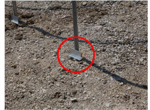
20. Attach Bottom Wood Adapter Brackets
