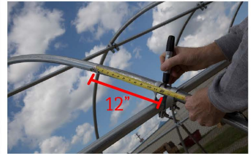
16. Install Side Braces 12" From Top Of 5' 2" Arch Frame
