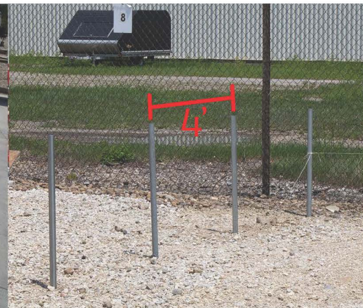
8. Measure & Line Up Support Posts 4' On Center
