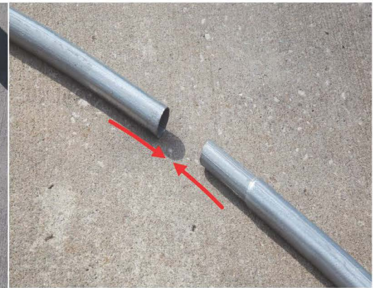
4. Connect Swedge Ends Together
