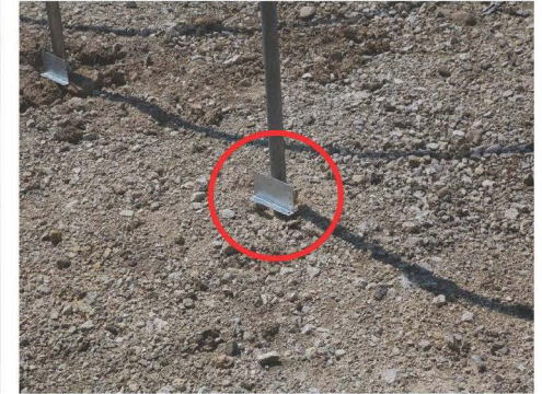
20. Attach Bottom Wood Adapter Brackets
