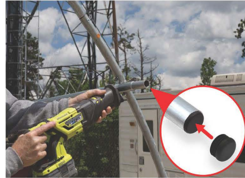
19. Cut Off Excess & Insert End Plug
