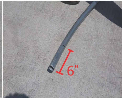
3. Confirm 6" Marks On Support Post
