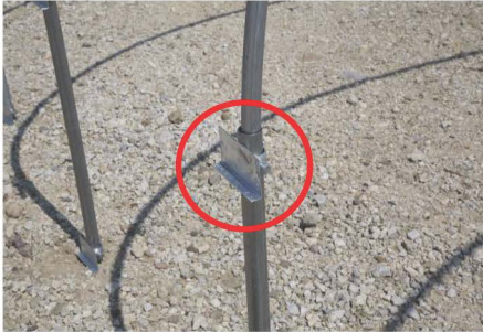
13. Attach Top Wood Adapter Brackets
