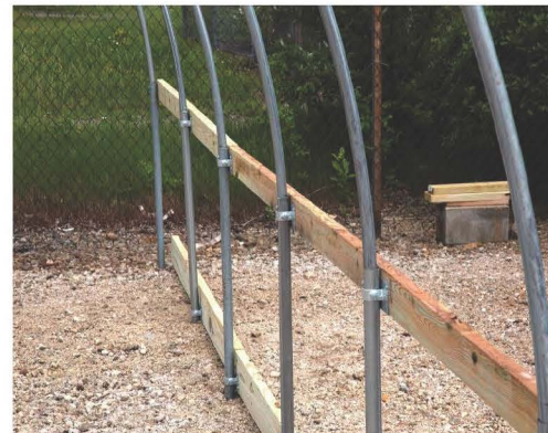
23. Finish Attaching Side Rails On Top & Bottom For Both Sides
