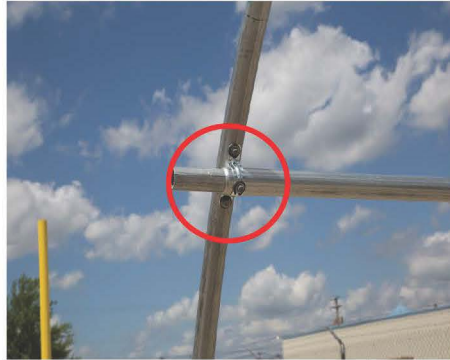
18. Use Pole Strap For Ends Of Side Purlin
