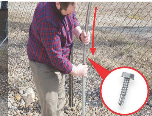
11. Slide Hoop In Support Post To 6" Mark & Connect Using Tek Screw
