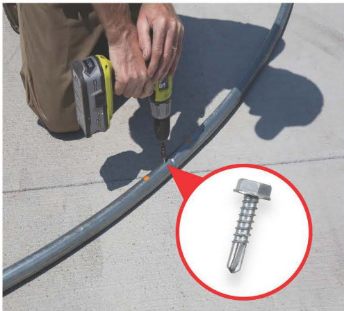
5. Use Tek Screw To Join Ends
