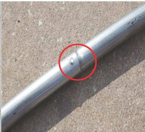
6. Confirm Connected Ends Are Secure
