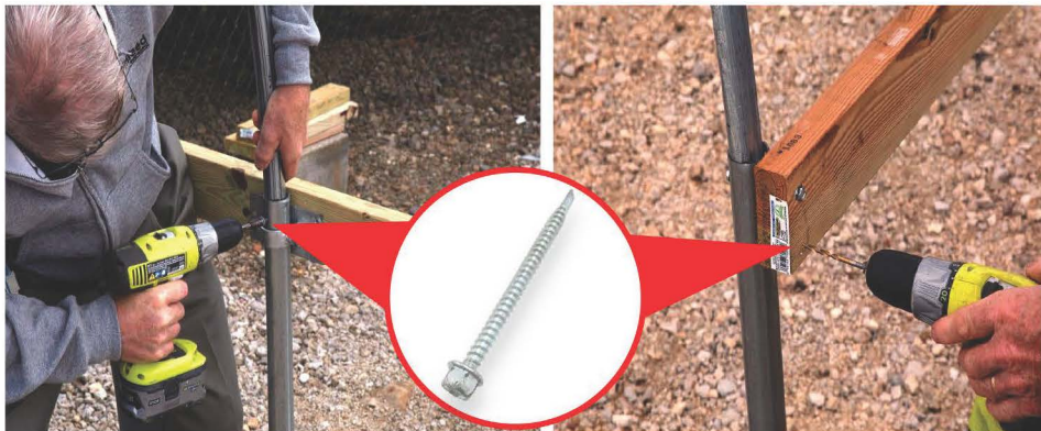
21. Attach Wooden Side Rails
