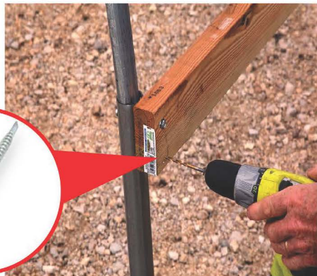
22. Screw Side Rails Into End Post
