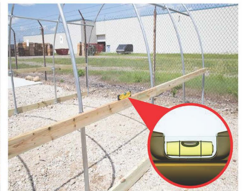
24. Make Sure Side Rails Are Level
