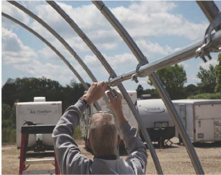
17. Finish Installing Side Braces For Both Sides
